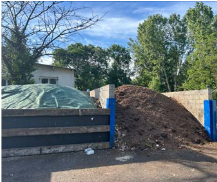
Figure 2 - Plateforme de compostage (Toilettes & Co)
