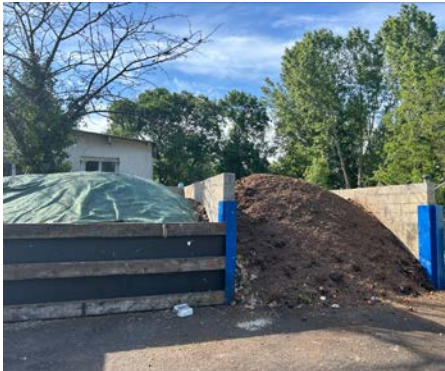
Figure 2 - Plateforme de compostage (Toilettes & Co)
